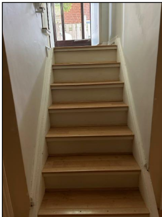
Missing handrail
