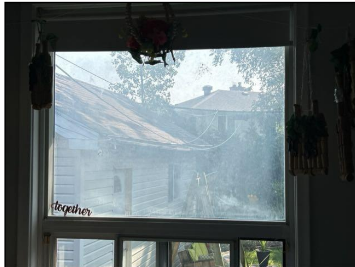
Lost seal on double or triple glazing
