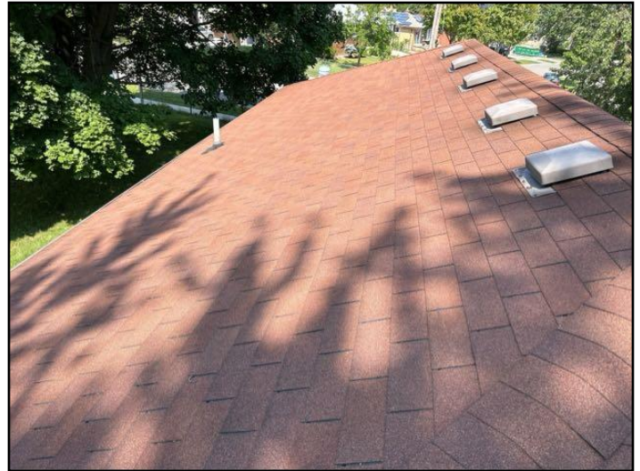
Asphalt shingles
