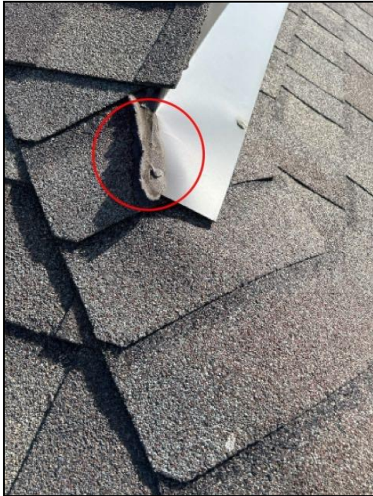
Loose flashing
