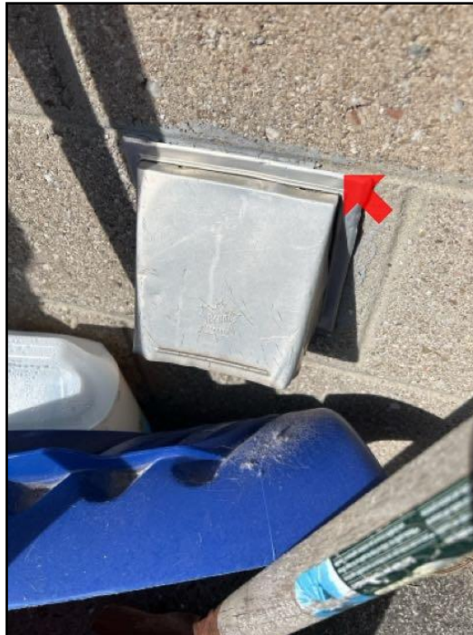
Caulking deteriorated/missing
