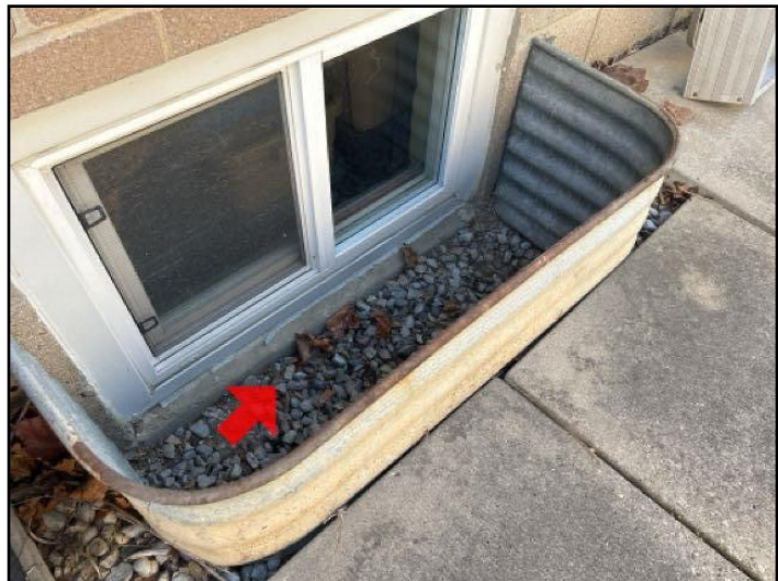
Less than 6 inches below window
