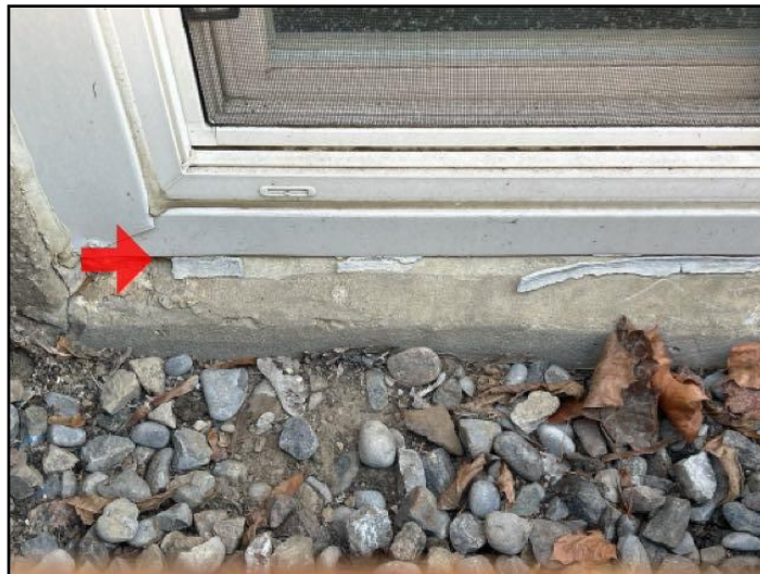
Caulking missing, loose or deteriorated
