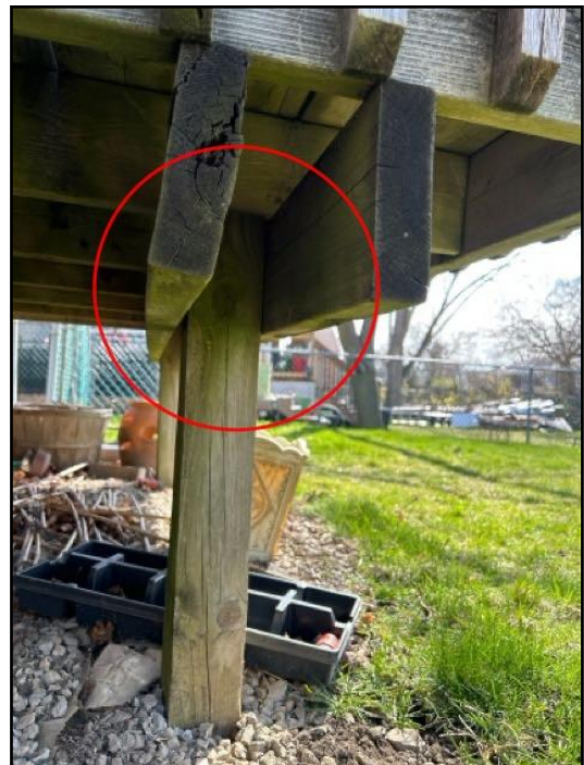
Poor connection/bearing
