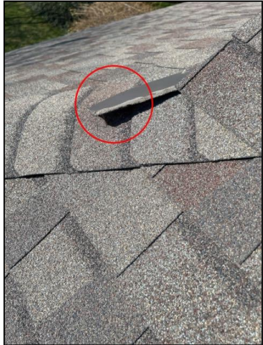
Loose flashing
