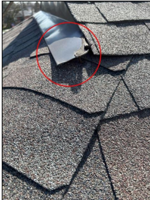
Loose flashing
