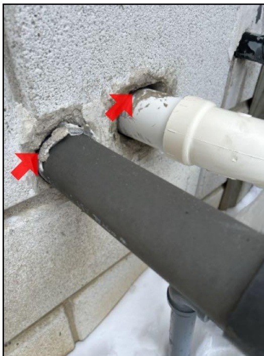
Caulking deteriorated/missing
